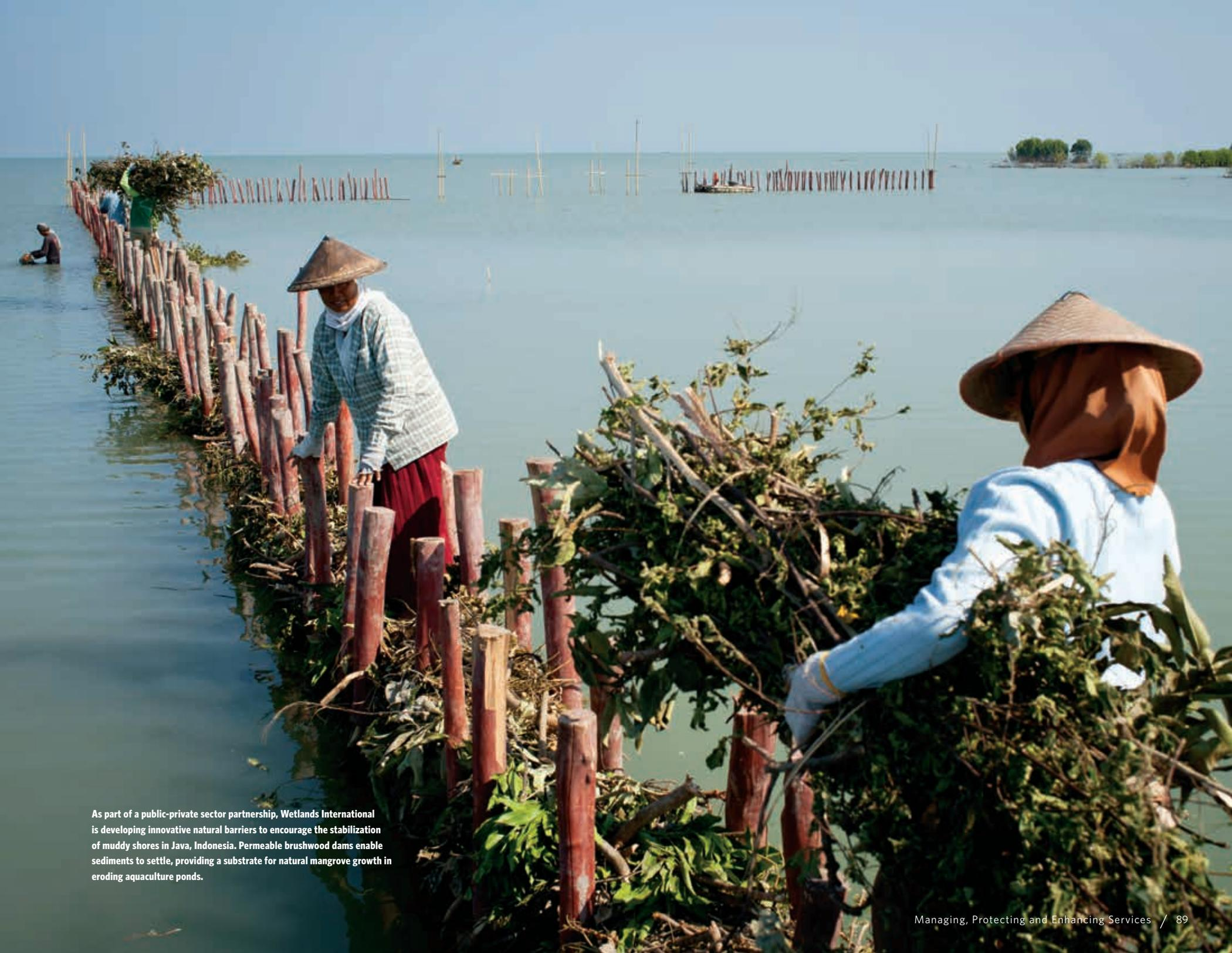
As part of a public-private sector partnership, Wetlands International is developing innovative natural barriers to encourage the stabilization of muddy shores in Java, Indonesia. Permeable brushwood dams enable sediments to settle, providing a substrate for natural mangrove growth in eroding aquaculture ponds.
